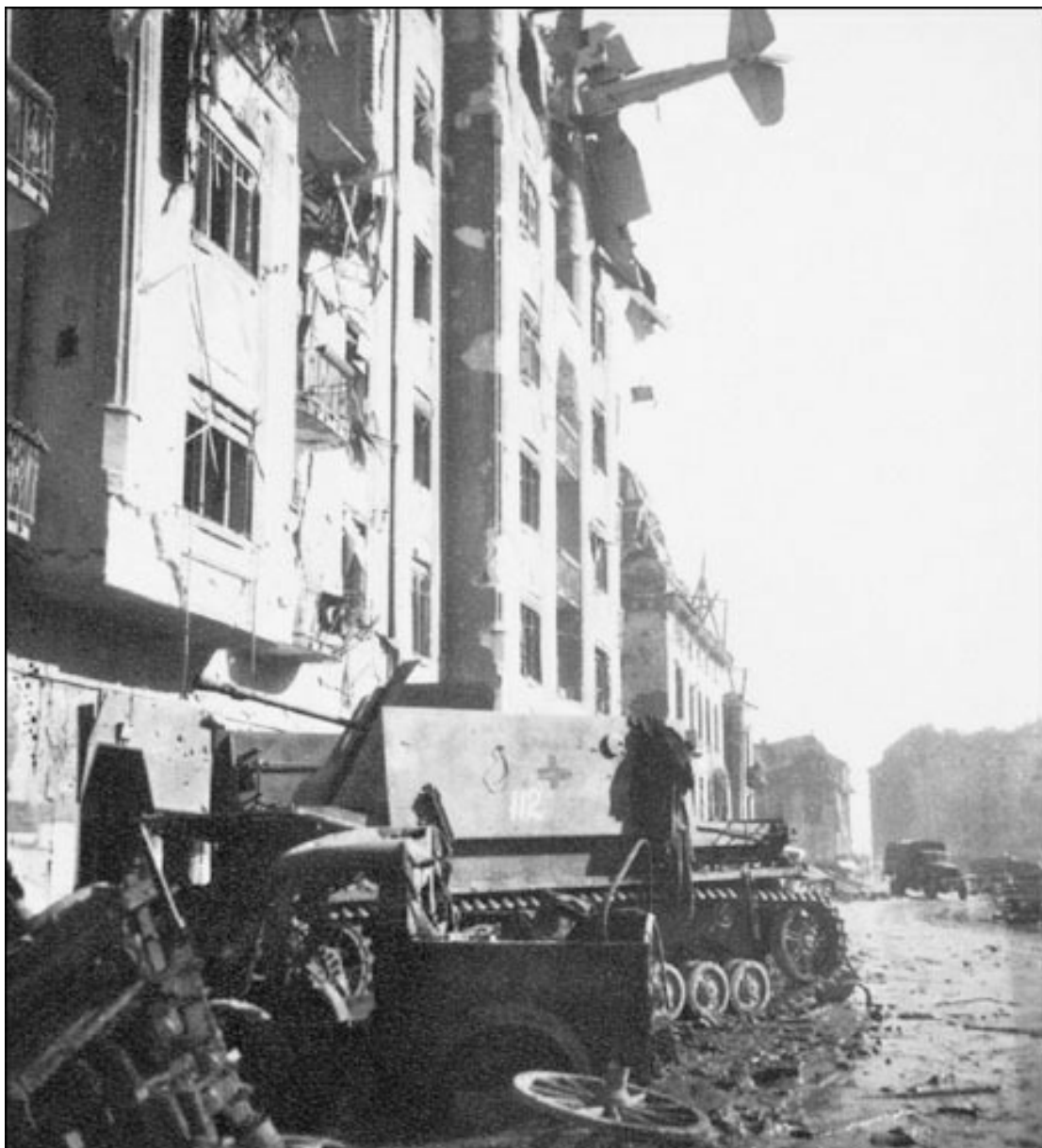
A German Flakpanzer IV abandoned on a Budapest street. In the background, a German glider that has crashed into the wall of a building is visible. These gliders were used to bring in supplies to the city's garrison.
