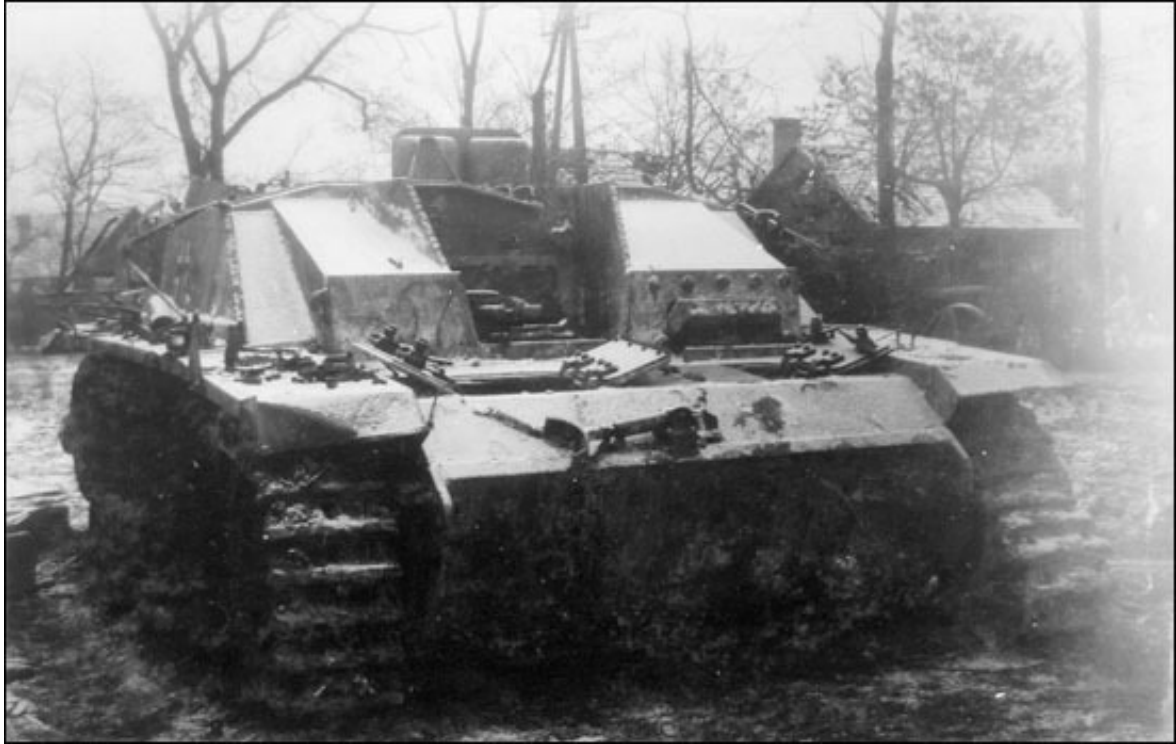
A StuG III self-propelled gun with its gun removed. Most likely, this machine was abandoned and cannibalized for its useful parts in order to repair other StuG IIIs.
