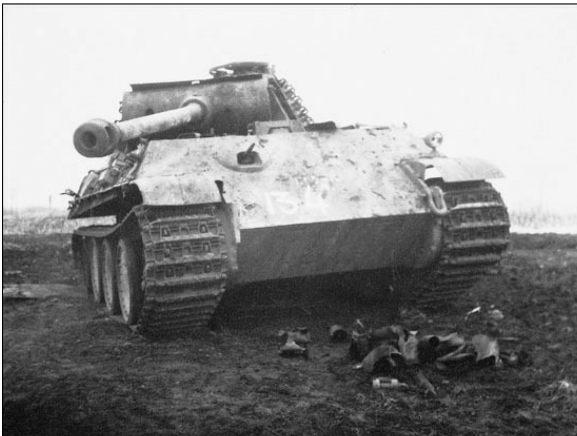
A German Panther Ausf.G with the number "134", given to it by the Soviet inspection team. The tank has no visible damage. Probably it was abandoned by the crew after experiencing mechanical problems.
