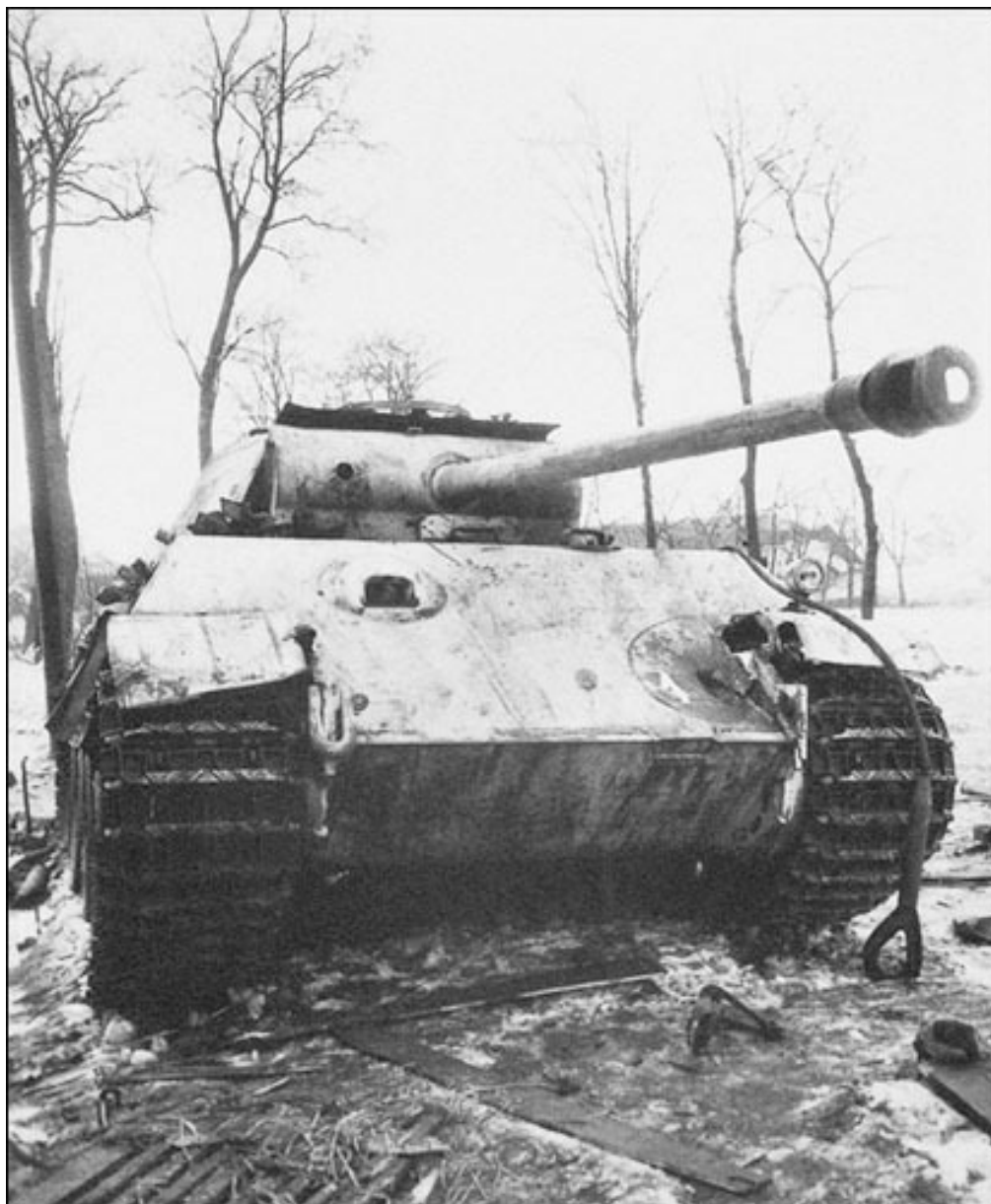
A knocked-out German Panther tank. The penetrating shell hole is clearly visible in the upper forward armor.
