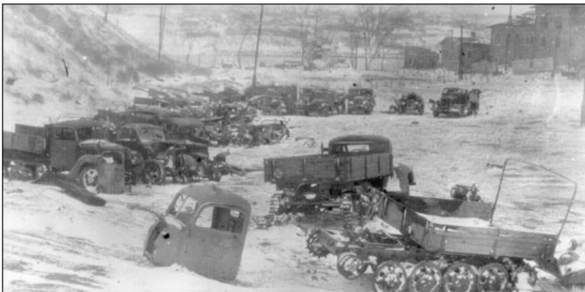
A graveyard of German equipment in Budapest. In the foreground are two disassembled RSO (Raupenschlepper Ost) fully tracked prime movers. (TsAMO)
