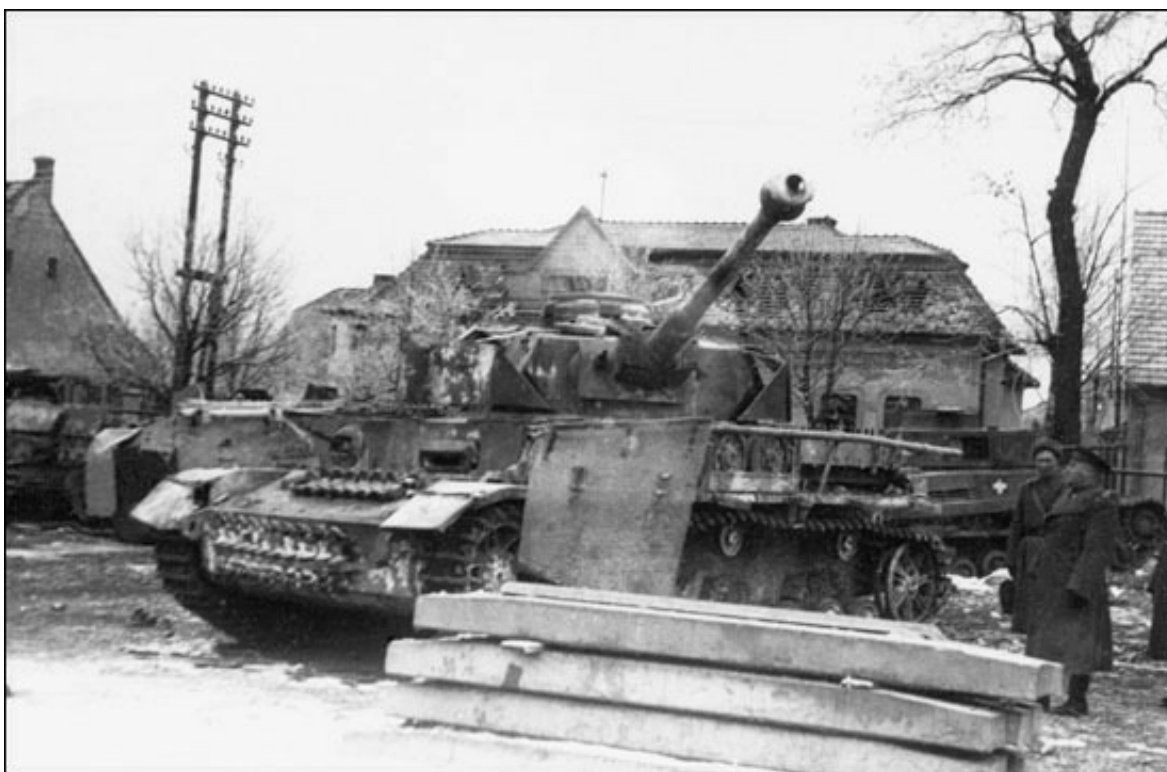
Soviet officers examining a Pz.IV tank, abandoned on a street of a Hungarian town. Note the tank's Schürzen armored skirting, designed to protect the tank against anti-tank rifle rounds and hollow-charge shells.
