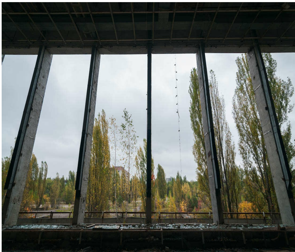
The Palace of Culture's main hall windows
