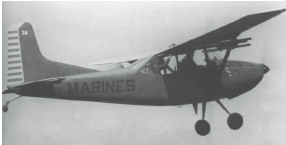
Cessna O-1 Bird Dog, a light single-engine observation and air control air -craft. The Bird Dog was in the Marine Corps inventory from World War II through Vietnam.
