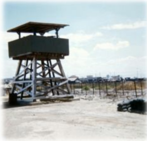
One of many elevated bunkers at Bien Hoa Airport.
